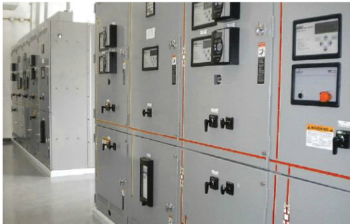
Paralleling switchgear at Columbus Regional Healthcare runs routine power system testing and energy management during peak periods.
