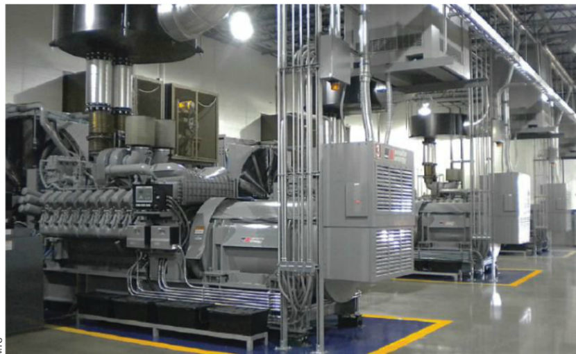
Four 2,500-kW gensets at the Medical Regional Healthcare System, GA
