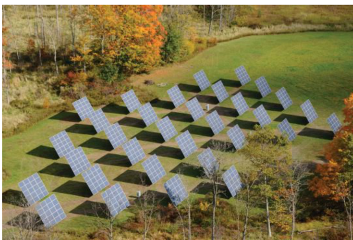
Thirty-nine-kilowatt solar installation
